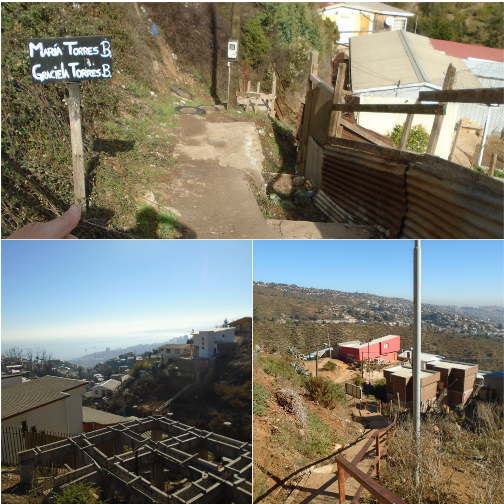
FIGURE 1 Places still unreconstructed 5 years after the fire because they are not part of the institutional plan
